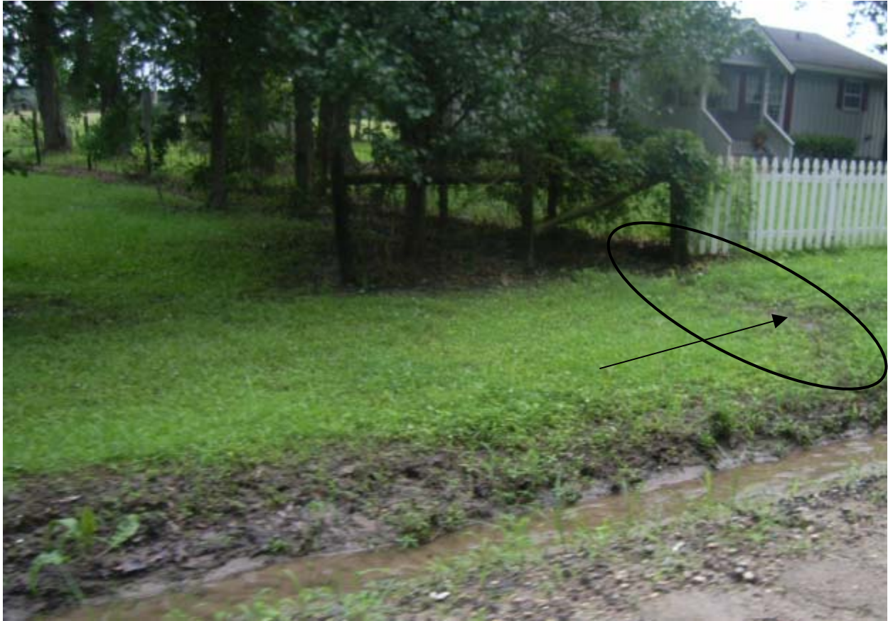
Figure 26. As seen in the photograph a trench that runs off to a road side storm water ditch. For preventing stormwater runoff from areas with pet waste or malfunctioning on site septic systems, planting of vegetative buffers or other BMPs are recommended.
