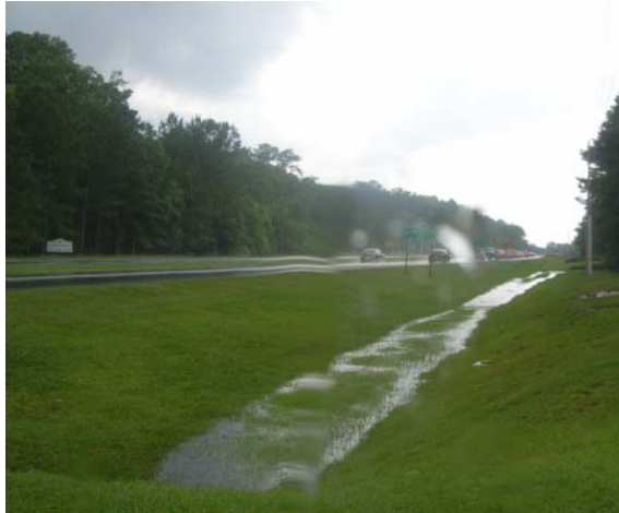
Stormwater ditch along US 278 following a scattered thunderstorm activity on June 8, 2009.
