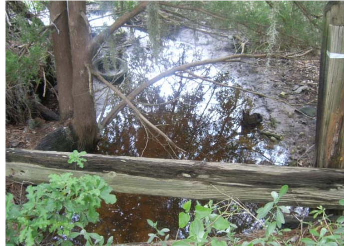
Road erosion and debris off of Pinckney Colony Road, flowing towards Okatie River
