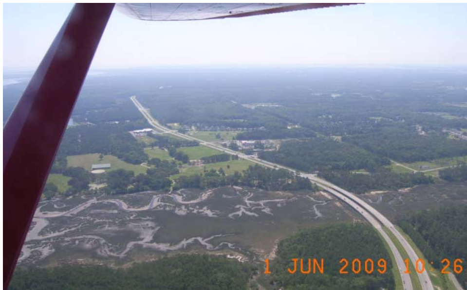
Figure 23: Aerial view of US 278 flying from west to east. Portion of the proposed widening of the US 278 is indicated on the picture Photograph was taken during low tide conditions.
