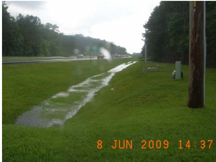
Figure 13. Stormwater ditch along US 278 within the Okatie River watershed. The photograph was taken following one of the localized scattered thunderstorm events on June 8, 2009.
