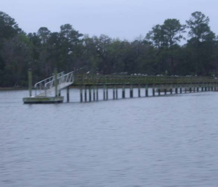
Birds on the railings of a private dock
