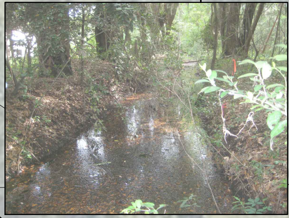
UPSTREAM FROM DITCH AREA FILLED WITH DIRT. WATER ELEV ~2.5' FROM DITCH BOTTOM, ESTIMATED WATER ELEV.=9.5'
