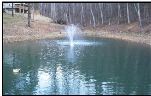
Figure 5. Collection pond with aeration fountain Photo courtesy of Rainwater Management Solutions
