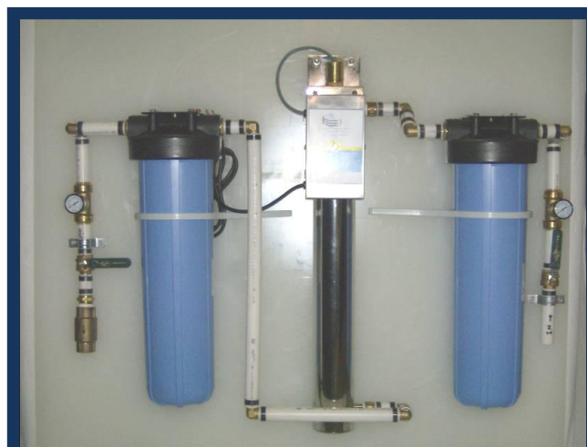
Figure 16. Water treatment system using a sediment filter, an ultraviolet light and a carbon filter.
