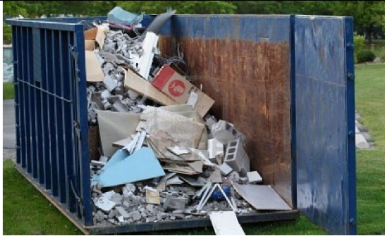
Construction waste and materials handling is part of any Stormwater Pollution Prevention Plan (SWPPP).
