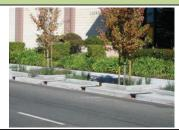
Tree Box Filters are containers filled with a soil mixture, a mulch layer, under-drain system and a shrub or tree similar to flow through planters. The compact size of tree box filters allow volume and water quality control to be tailored to specific site characteristics and are well suited to urban areas. Tree box filters provide the added value of aesthetics while making efficient use of available land for stormwater management.
