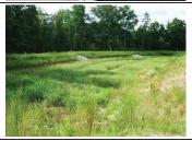
Dry detention ponds are basins whose outlets have been designed to detain stormwater runoff for some minimum time (e.g., 24 hours) to allow particles and associated pollutants to settle. Unlike wet ponds, these facilities do not have a large permanent pool of water. However, they are often designed with small pools at the inlet and outlet of the basin. They can also be used to provide flood control by including additional flood detention storage.
