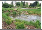
Wet Detention Ponds. The pond consists of a permanent pool of water into which storm water runoff from each rain event is detained and treated in the pond until it is displaced by runoff from the next storm. Sedimentation processes remove particulates, organic matter, and metals, while dissolved metals and nutrients are removed through biological uptake.
