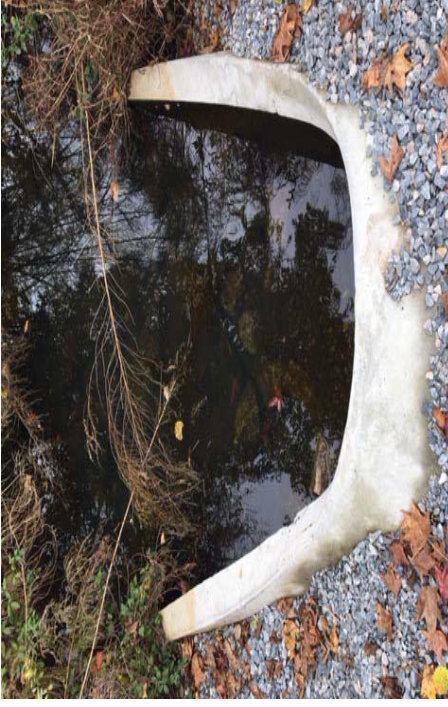
WMPOut: N32.260125 -80.857240 Sampling point for water exiting wet detention pond into vegetated wetland
