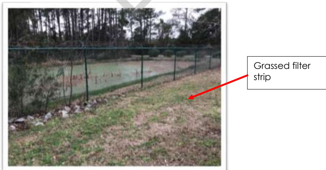
Figure 14. St. Helena – Wet pond on the south side of site, outside fence
