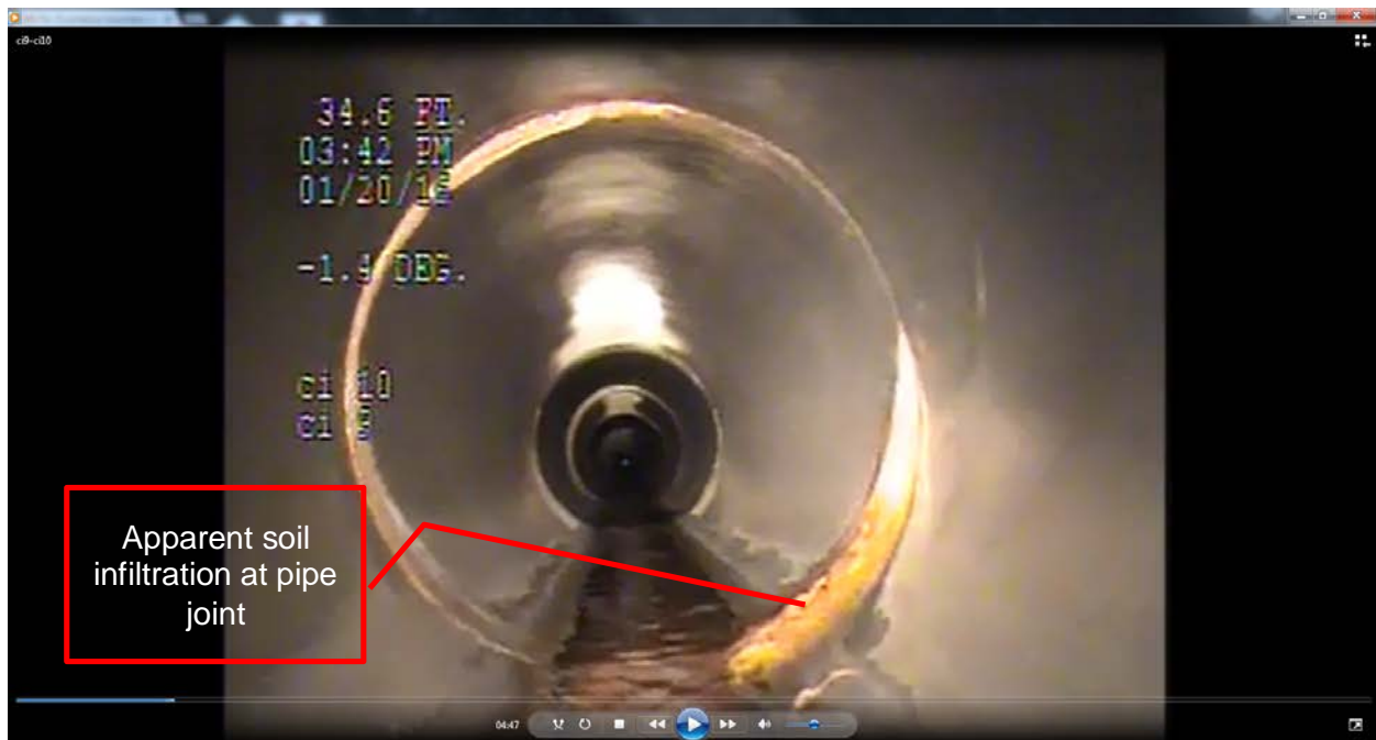
Figure 13: Pipe CI9-CI10: Sediment accumulation at pipe joint likely from infiltration through joint.
