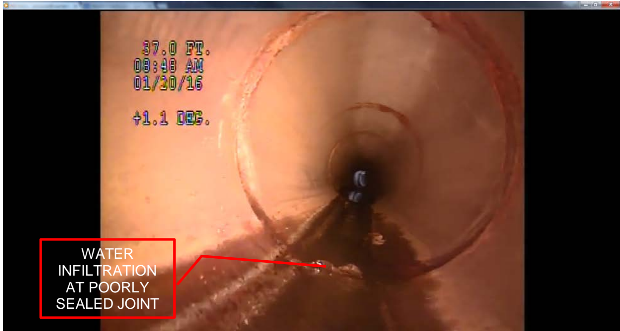
Figure 7 - Pipe C15-C16: Evidence of water infiltration through pipe joints
