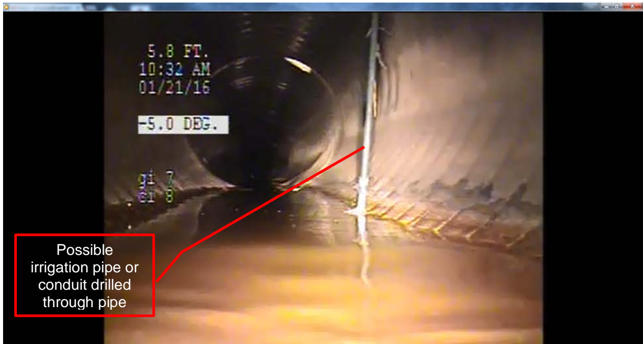
Figure 11: Pipe GI7-GI8: Irrigation pipe or electrical conduit drilled through pipe.
