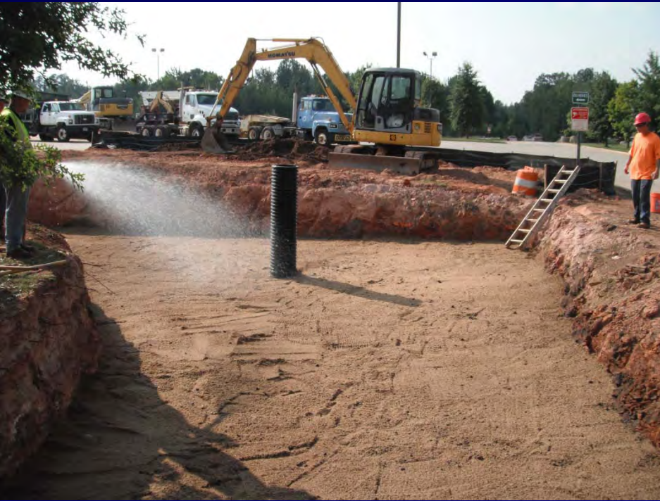
Installed engineer soils in 1 ft lifts and watered to consolidate.
