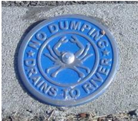
Placards found on storm drains and catch basins.
