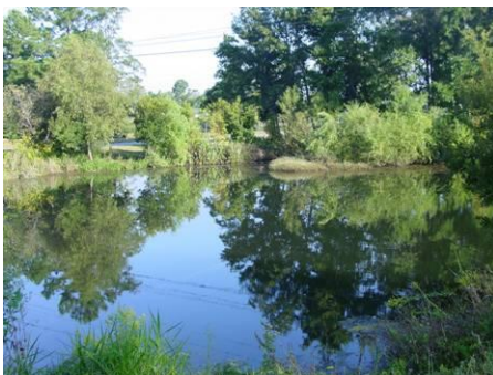
Landscaped stormwater retention basin.
