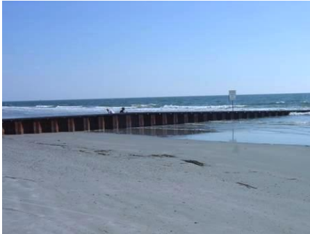
A portion of Hunting Island's beaches were renourished in 2006 and groins were installed.
