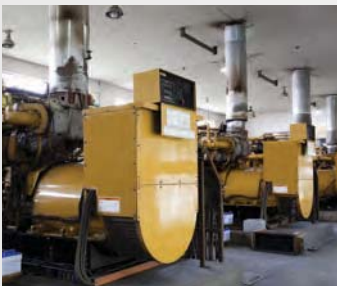
Emergency Generator Battery Charging
