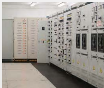
Reliable Switchgear Power
