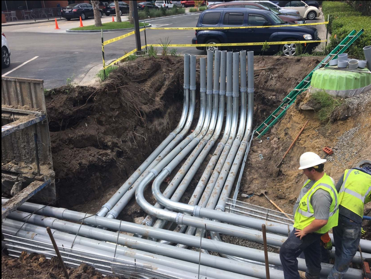
Duct bank at Palmetto & Boundary Street. Duct Bank construction is 90% complete.
