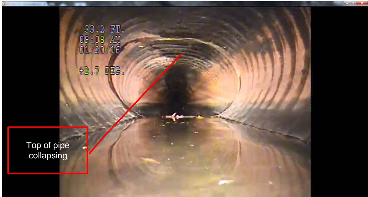
Figure 9: Pipe CI5-JB2: Severe deflection such that pipe is beginning to collapse.
