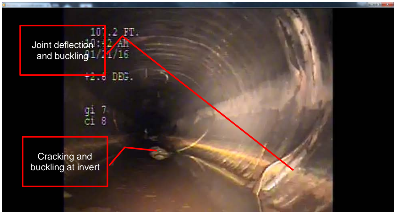
Figure 12: Pipe GI7-GI8: Joint damage likely from improper installation.
