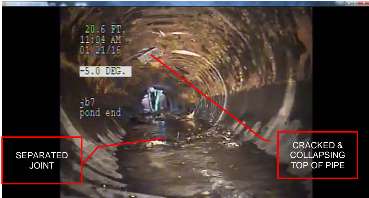
Figure 10: Pipe G17-PONDEND: Severe joint deflection and damage likely resulting during improper installation.
