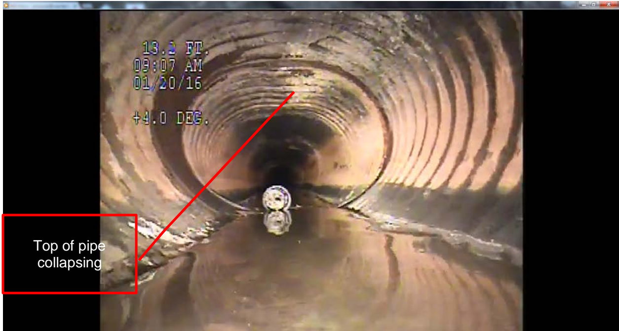
Figure 8 - Pipe CI5-JB2: Severe deflection and buckling beyond allowable limits
