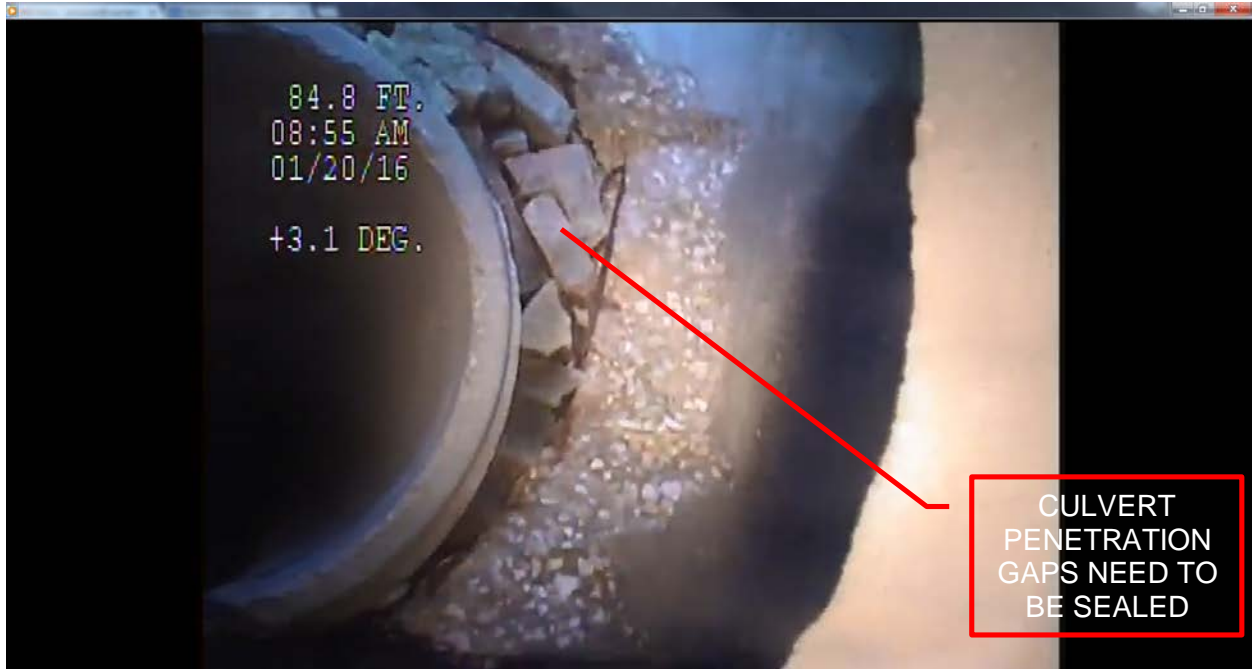
Figure 1 - Example of culvert penetration needing to be sealed with new grout.
