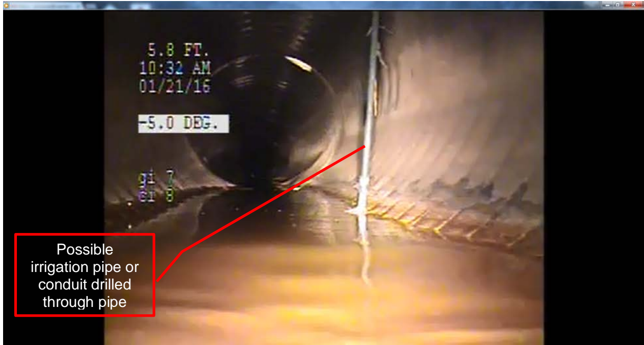
Figure 11: Pipe GI7-GI8: Irrigation pipe or electrical conduit drilled through pipe.
