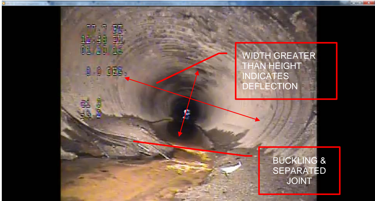
Figure 2 – Pipe JB2-C13: Pipe is experiencing sever deflection and joint separation/buckling
