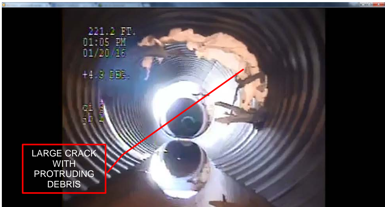
Figure 5 - Pipe JB2-CI3: Large cracks with debris penetration.
