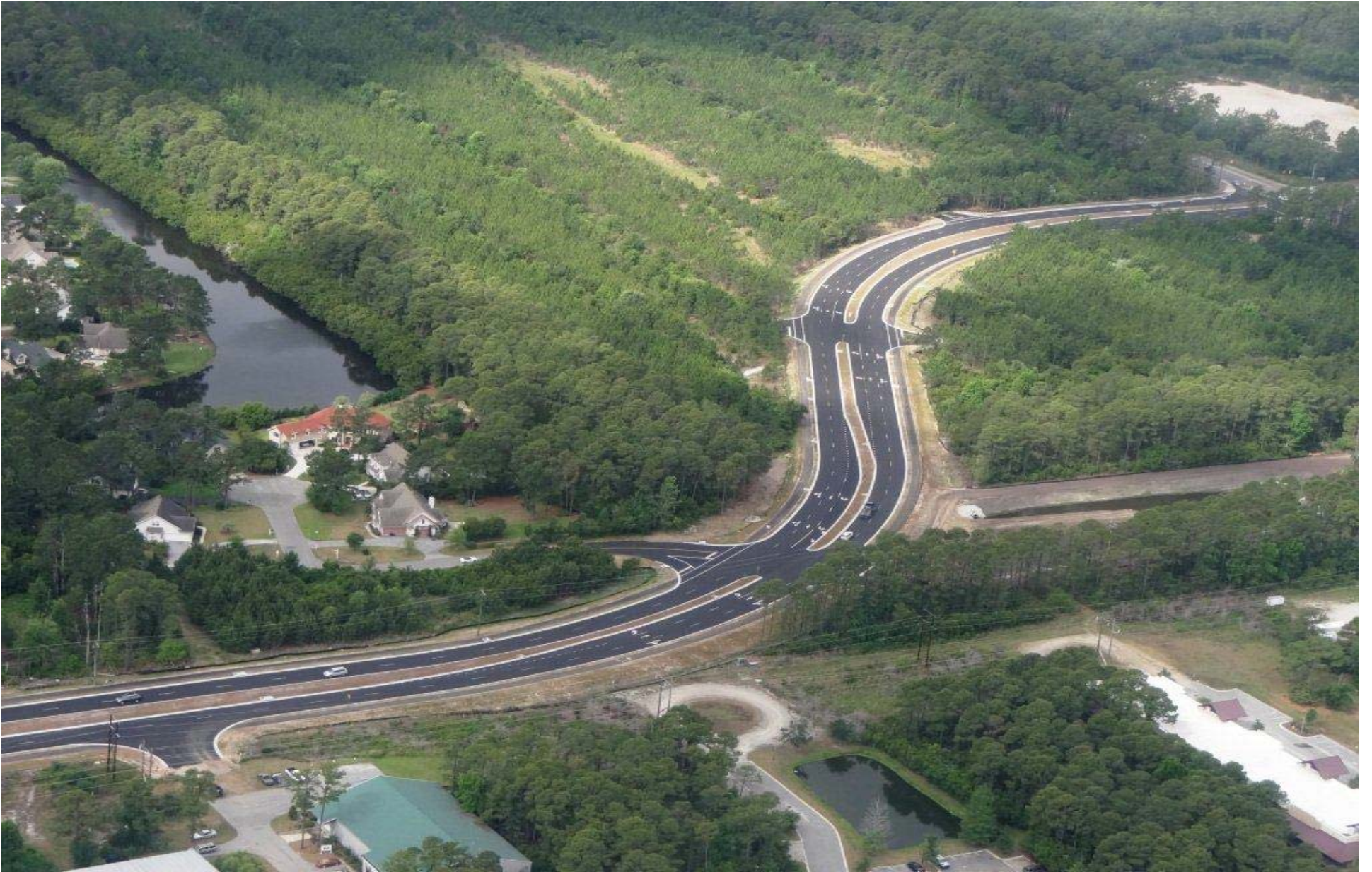
BLUFFTON PARKWAY PHASE 5A SEGMENT 1
