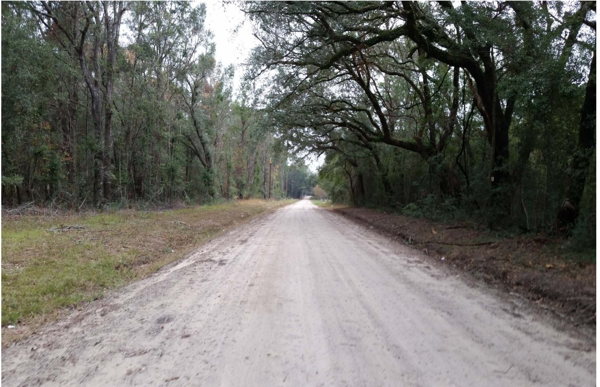
COUNTY DIRT ROAD BEFORE PAVING – WIMBEE LANDING ROAD
