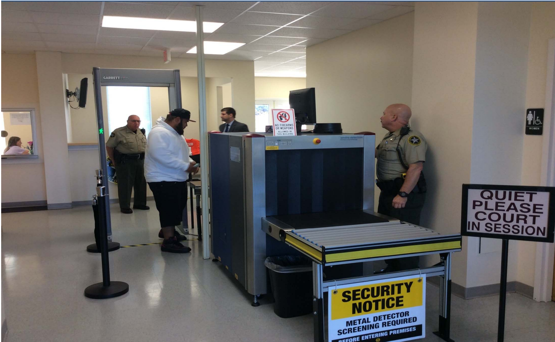
2 nd Floor Security Station – X-ray Unit, Walk Through Magnetometer and Door Strike/Card Access System
