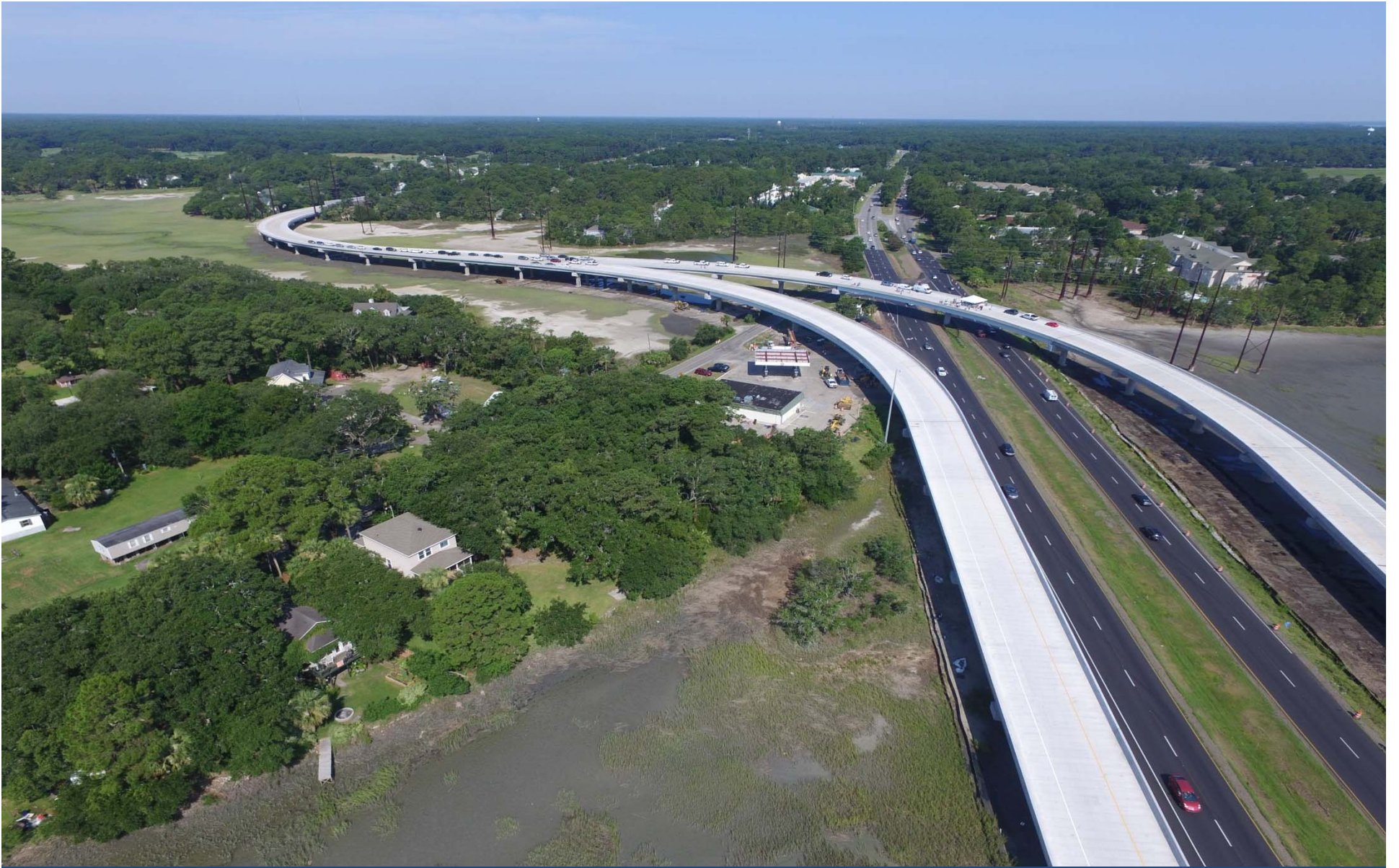
BLUFFTON PARKWAY PHASE 5A SEGMENT 2
