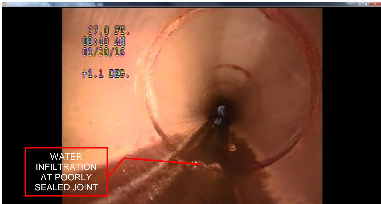
Figure 7 - Pipe C15-C16: Evidence of water infiltration through pipe joints
