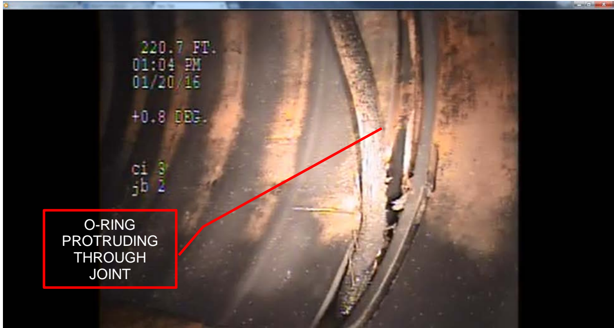
Figure 4 - Pipe JB2-CI3: Example of pipe joint failure with rubber gasket out of place.
