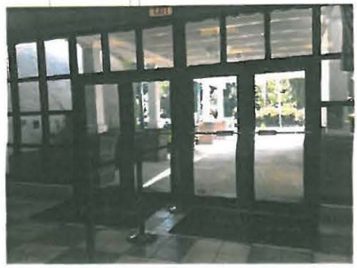
EXISTING Inside View of Main Building Doors
