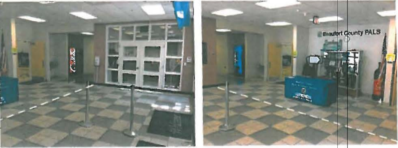
EXISTING Lobby with demarcation line for NEW Inside Lobby Doors
