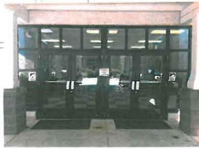
EXISTING Outside View of Main Building Doors
