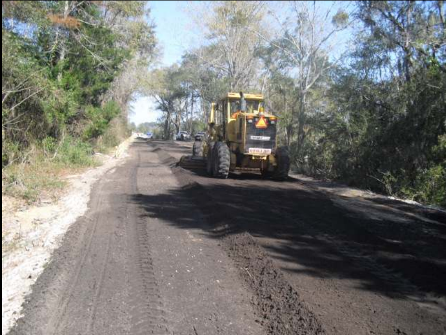
Final Grading of Access and Parking Area
