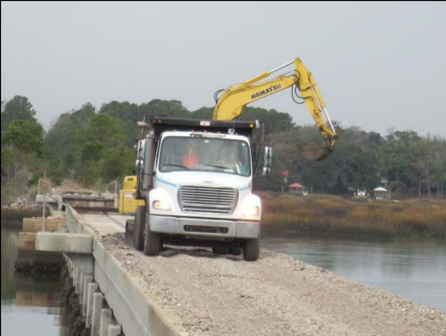
Removing Ballast Stone
