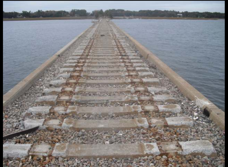
Ballast Stone and Concrete Crossties
