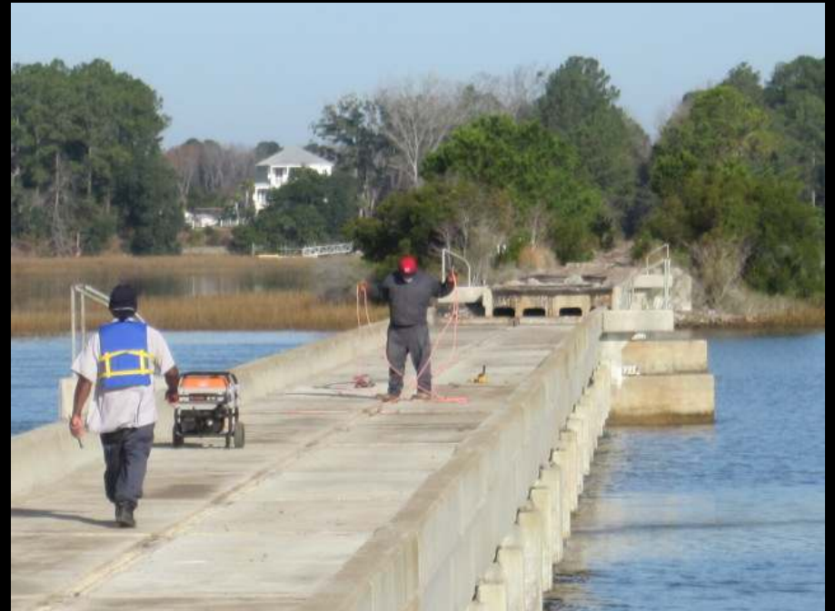
Preparing Pier Surface
