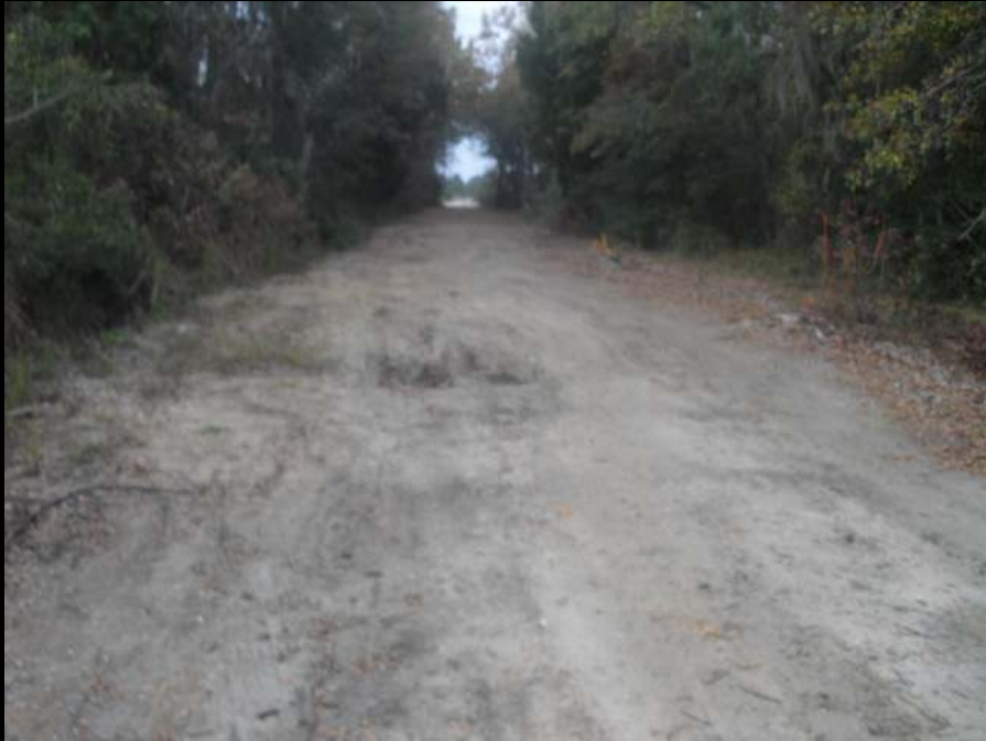
Approach from Seabrook Road
