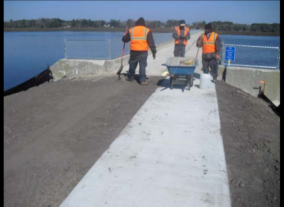
Mitigating Last Trip Hazard
