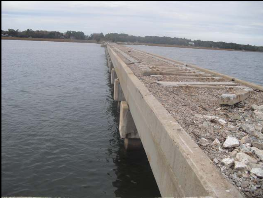
Foot of the Trestle
