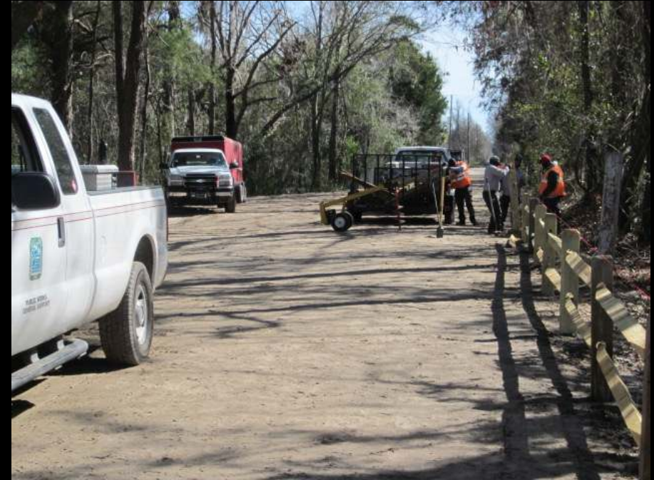
Installing Split Rail Fence
