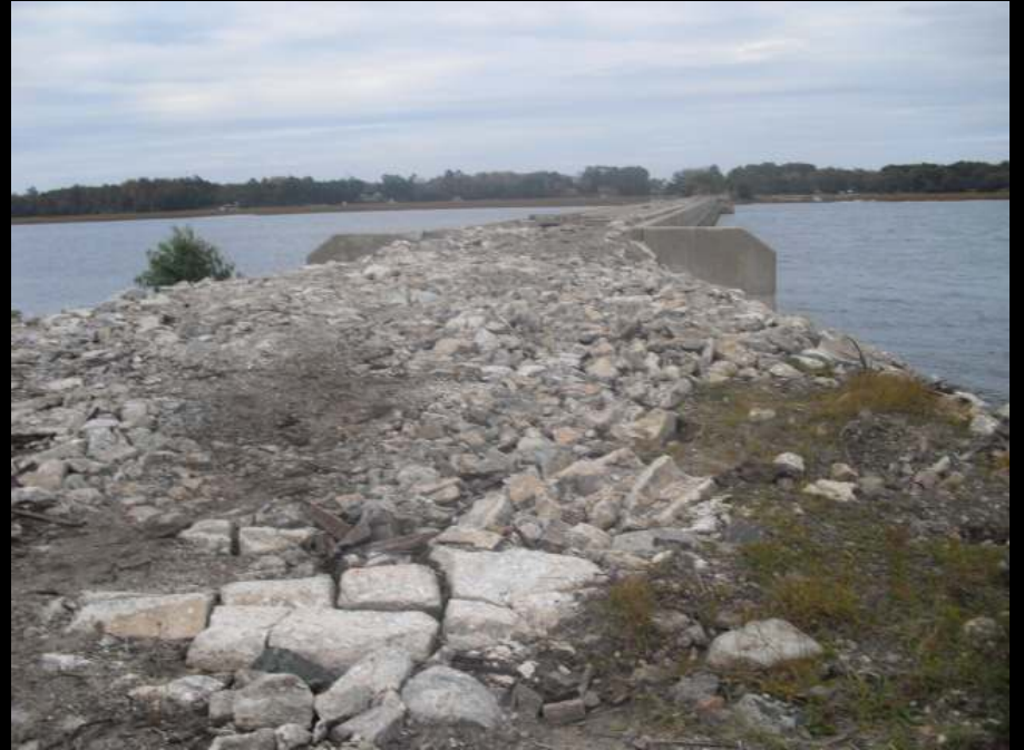
Foot of the Trestle
