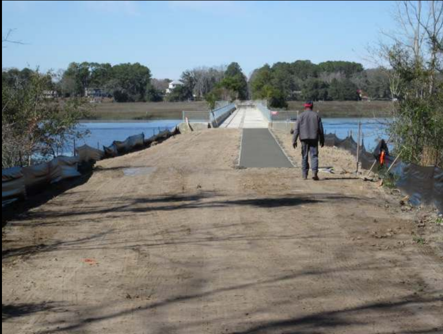
Newly Poured Handicapped Sidewalk; Safety Fencing Installed
