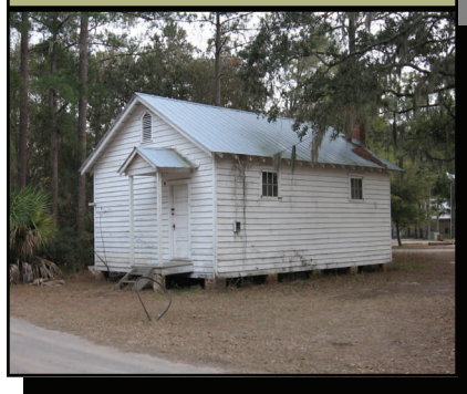
Old Schoolhouse restored as the Island's New Library.
