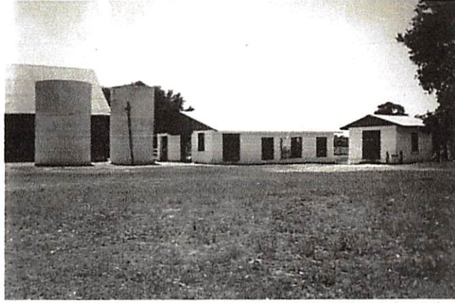
1940's with demolished barn to left, Sales House to right View of Silos
