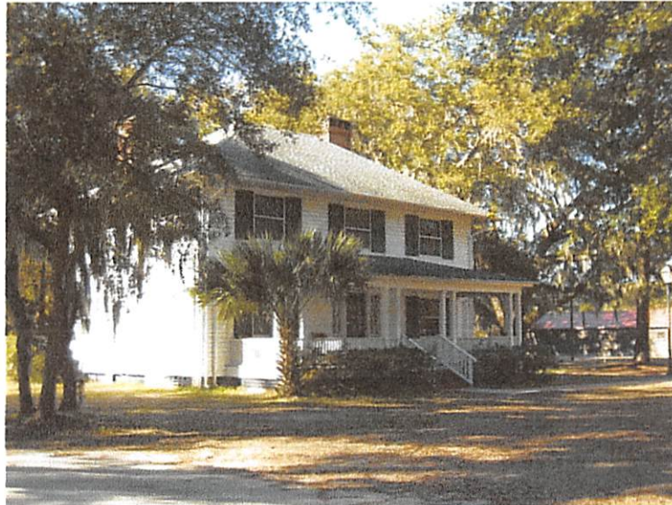
View of Front facing Dr. Martin Luther King Jr. Drive
