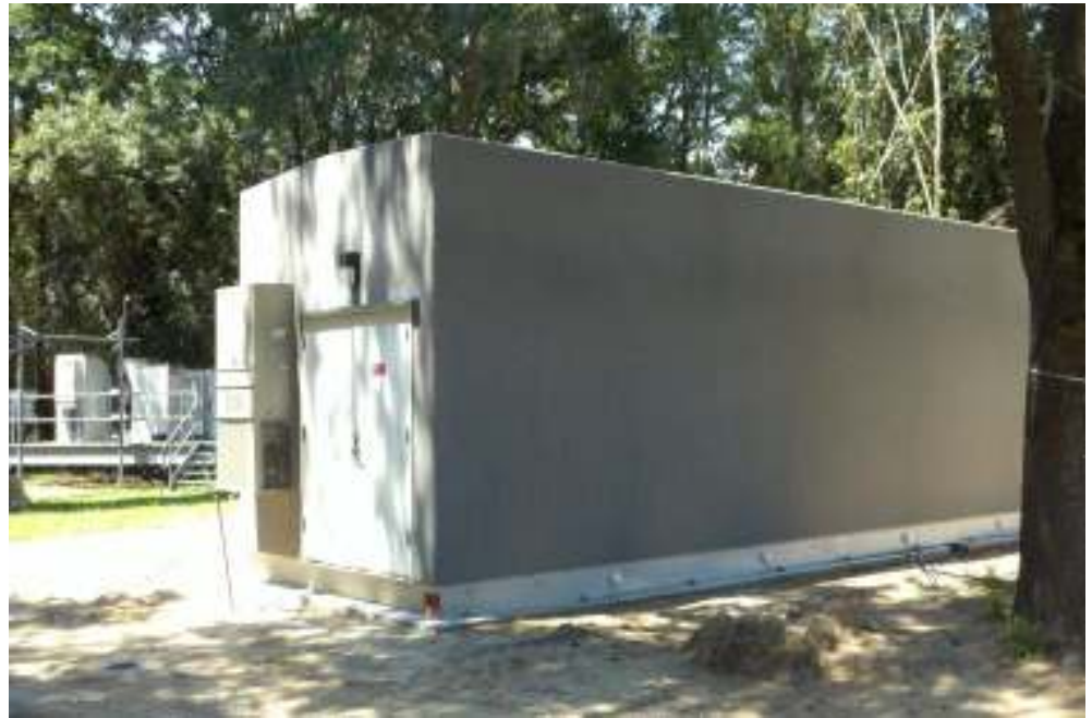
PSD Water Booster Station at Wildhorse Tower
