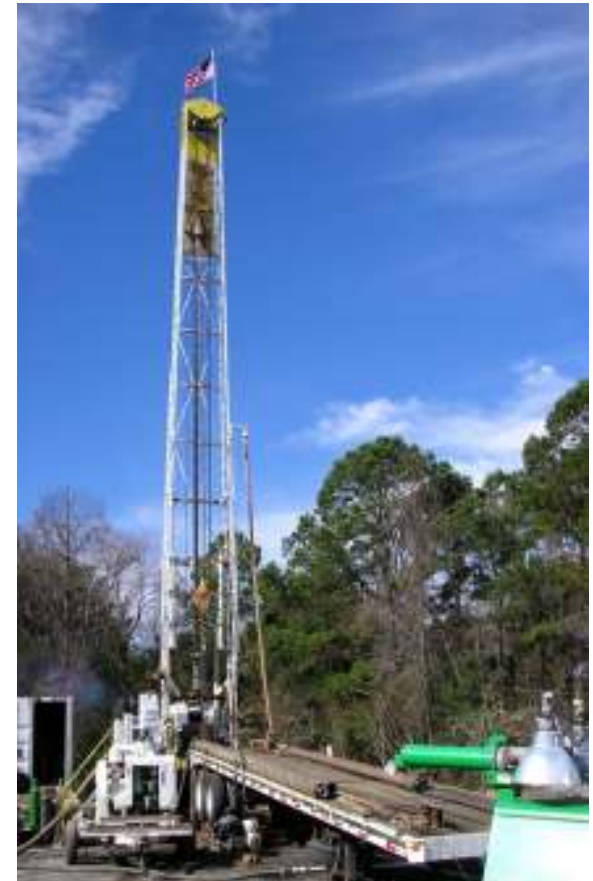
RO well drill rig
