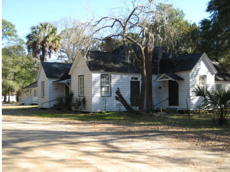
View of Front facing Penn Center Drive East
