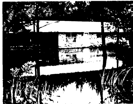
Residential Flooding - Causing property damage in many areas.
