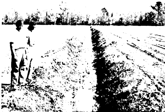
Lateral Canal - This canal shows importance of good construction, alignment, spoil management, and erosion control on side slopes.
