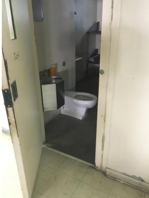
Existing Fixture in Cell
