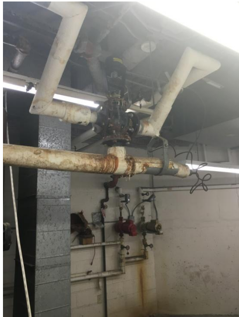
Existing Piping and Valve
