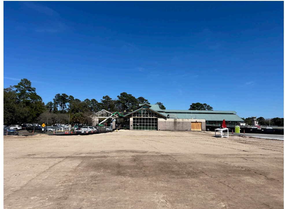
Mass Grading, Pad Prep
