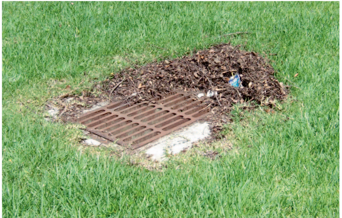
A result of leaf debris and litter buildup on a storm drain after a storm event. This drain needs to be cleaned as soon as possible.
