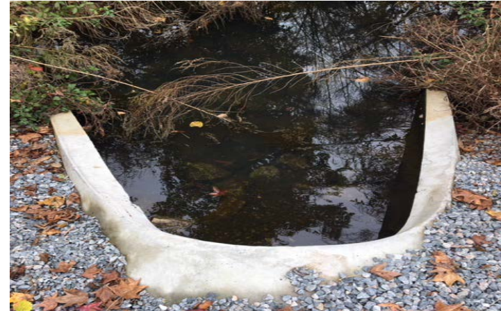
WMPOut: N32.260125 -80.857240 Sampling point for water exiting wet detention pond into vegetated wetland
