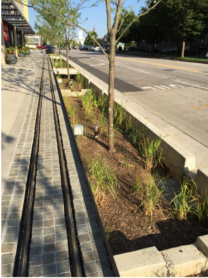
Figure 4.5. Example streetscape bioretention.
