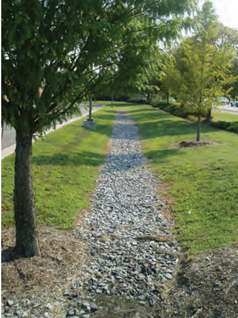
Figure 4.16. Infiltration practice in median strip.
