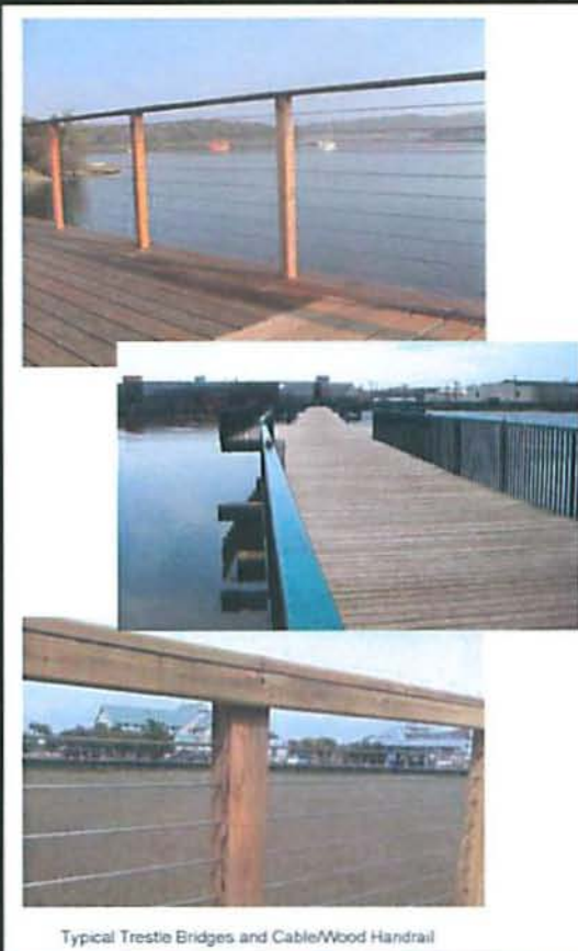
Typical Trestle Bridges and Cable/Wood Handrail
