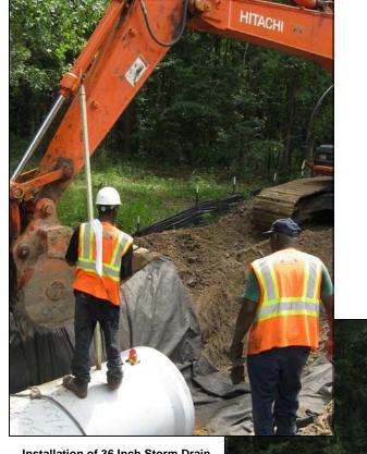
Installation of 36 Inch Storm Drain
