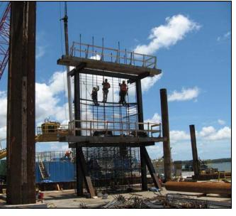
**Construction Workers Tying Rebar for Bridge Construction**
