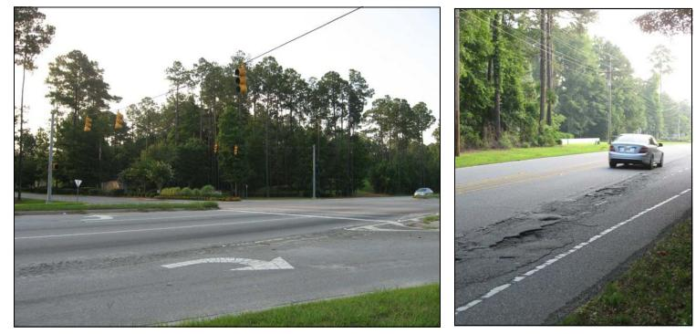
Alligator Cracking at the Intersection of Tide Watch Drive and SC 170
