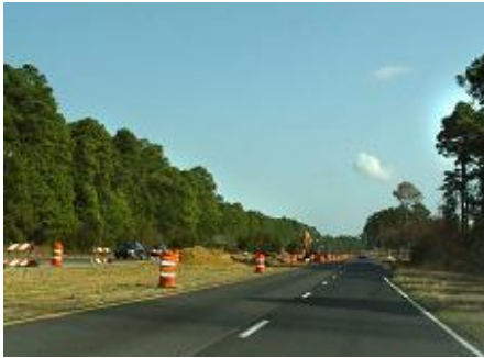
U.S. 278 was widened to six lanes between the Hilton Head Bridge to Simmonsville to increase capacity to accommodate existing and future traffic demands.
