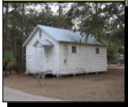
Old Schoolhouse restored as the Island's New Library.
