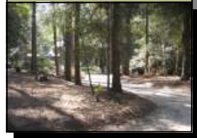
A sinking road
