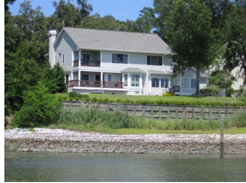
Image 10. An example of bulkheading along the May River.
