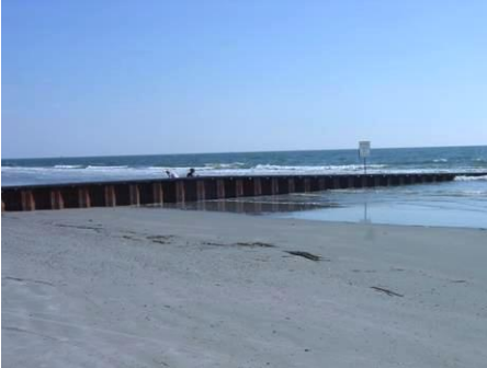
A portion of Hunting Island's beaches were renourished in 2006 and groins were installed.
