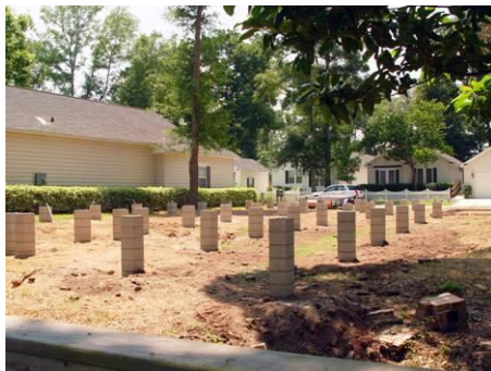
Only 24% of the County’s soils do not have severe limitations to the construction of dwelling units
