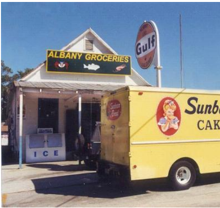
Albany Groceries, located in Dale, is a good example of commercial vernacular architecture.
