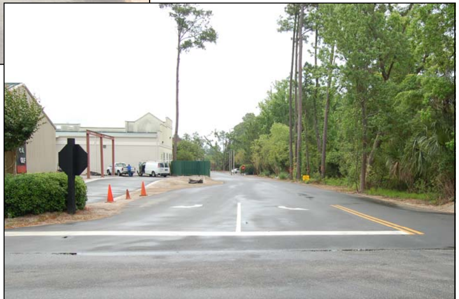
Completed Paving for New Frontage Road
