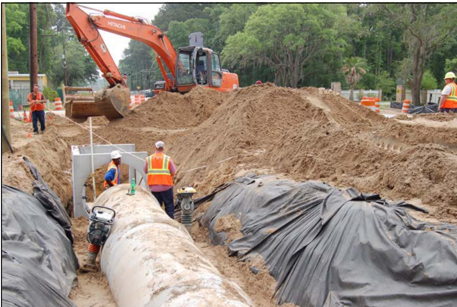
Installation of 42 Inch Storm Drain
