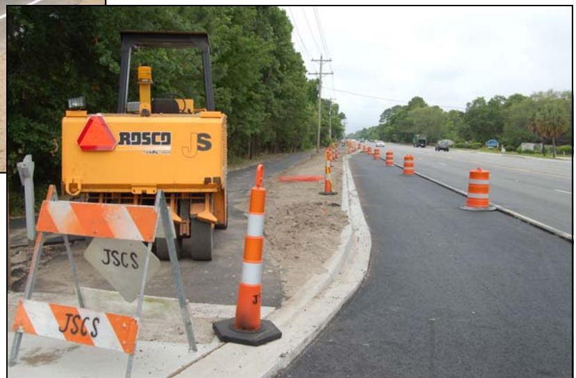
New Turn Lane from William Hilton Parkway to Burke's Beach Road
