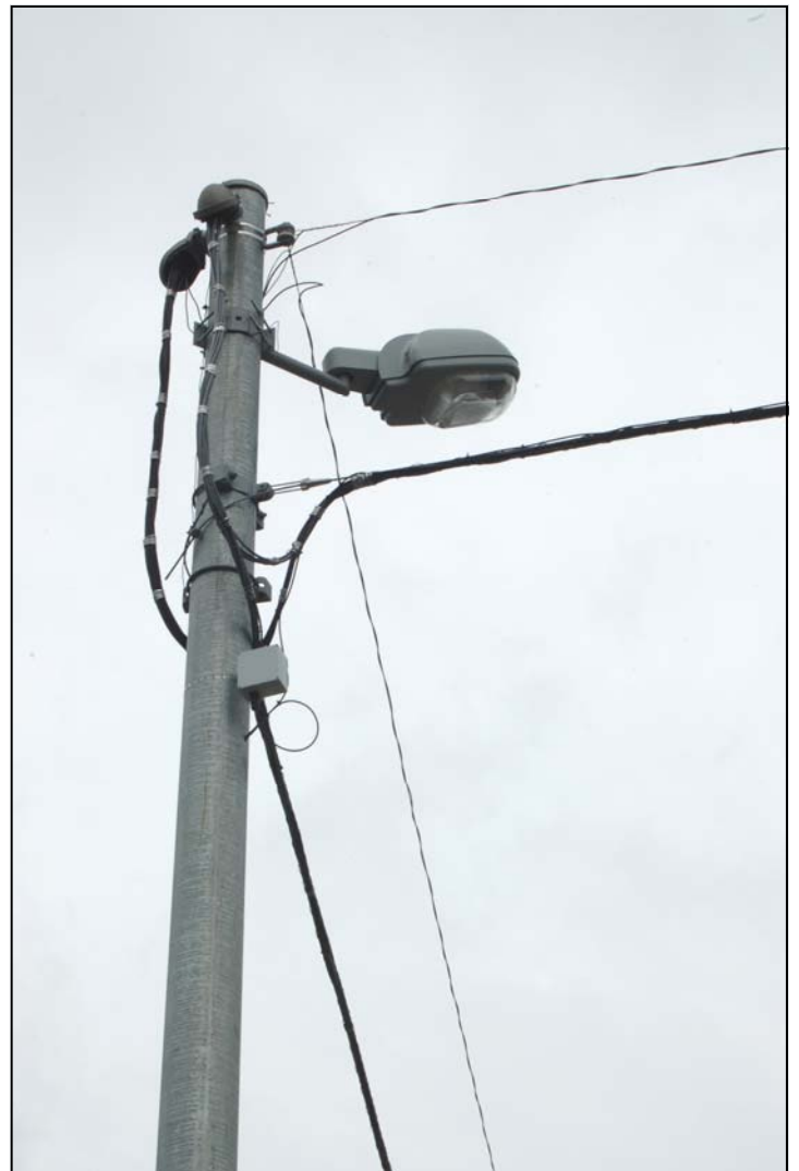
Detailed View of Newly Installed Street Light Fixture
