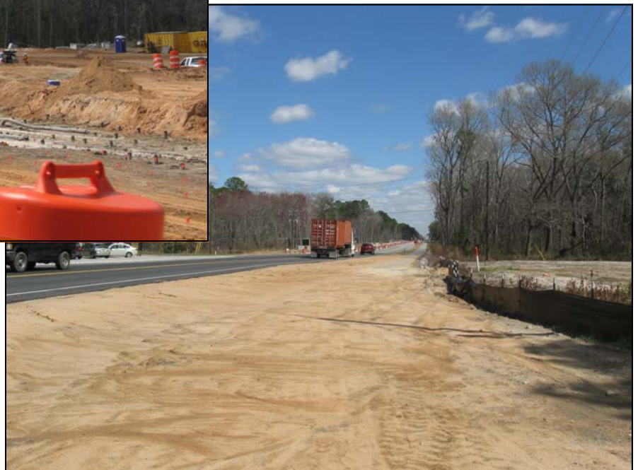
Embankment Build-up for Future Travel Lanes
