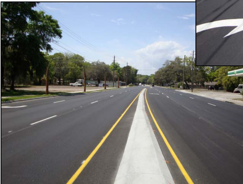
Concrete Paved Median
