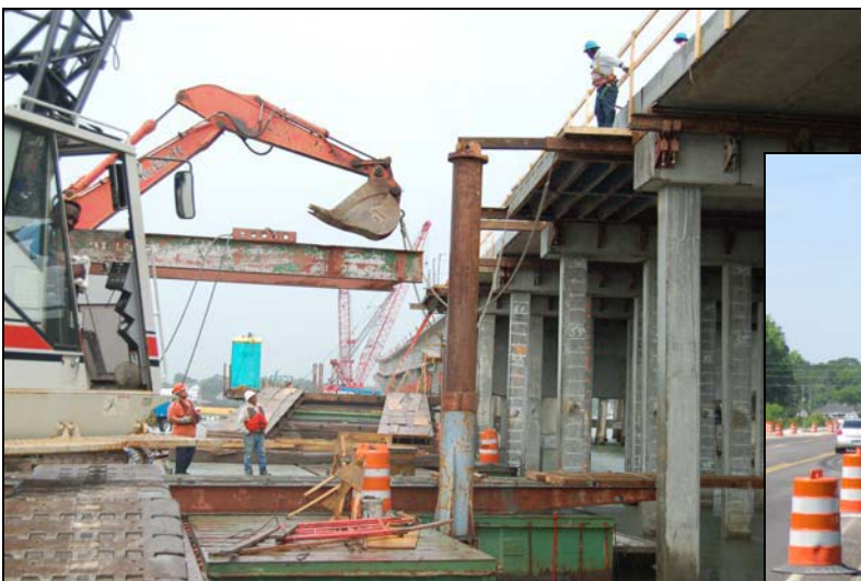
Bridge Crew Removing the Braces for the Poured Concrete Bridge Deck
