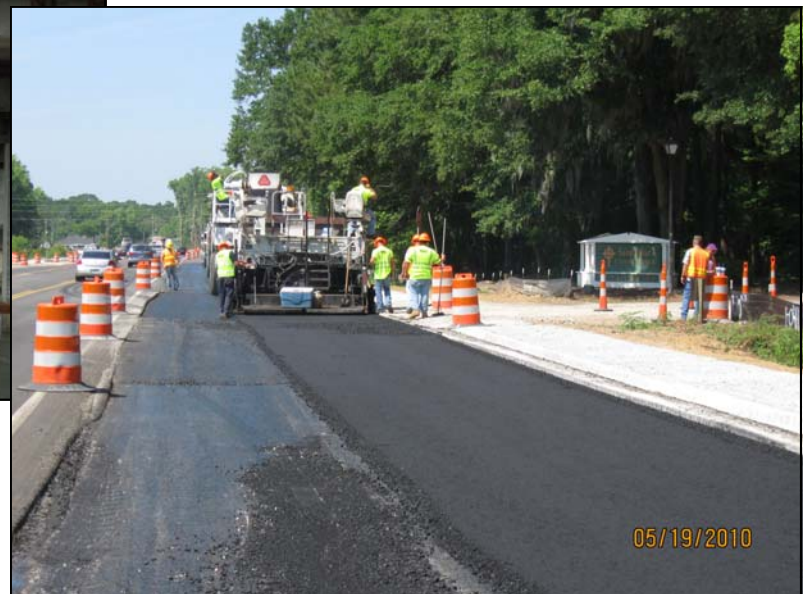
Installing Base Course Near St. Peter's Catholic Church
