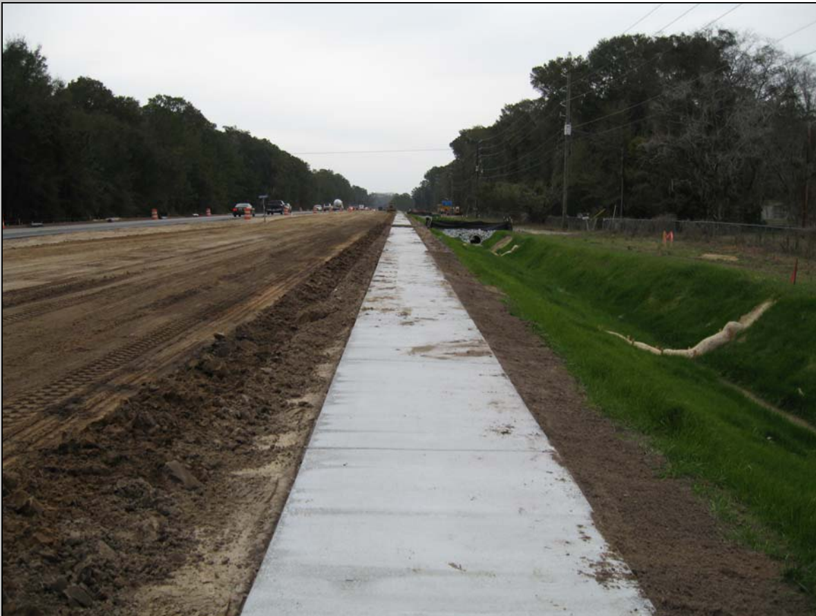
Finished Sidewalk on Lady's Island Drive
