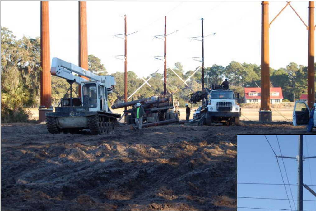
Santee-Cooper Moving New Power Poles into Place
