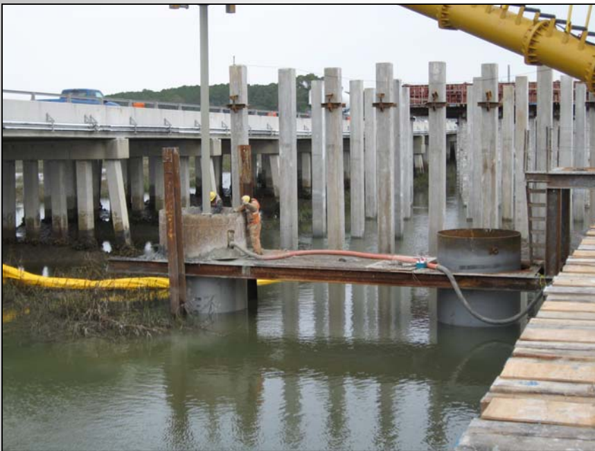
First Drilled Shafts on the East End of the New Bridge
