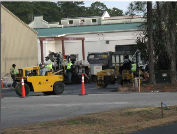
Paving Operations on New Frontage Road
