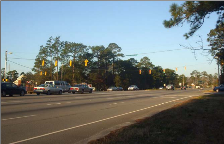
New Street Light Fixtures at the US 278 / Burnt Church Rd. Intersection
