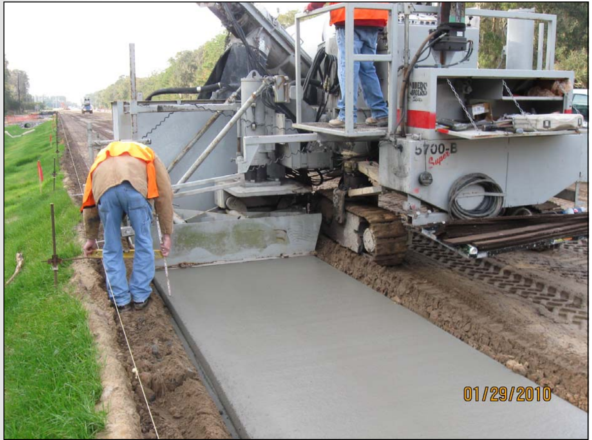
Placing Sidewalk on Lady's Island Drive
