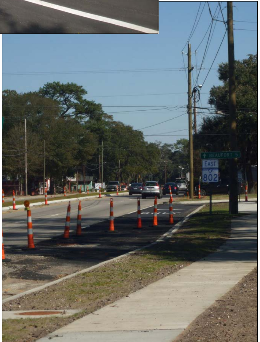
New Turn Lane from SC 802 to West Paris Avenue
