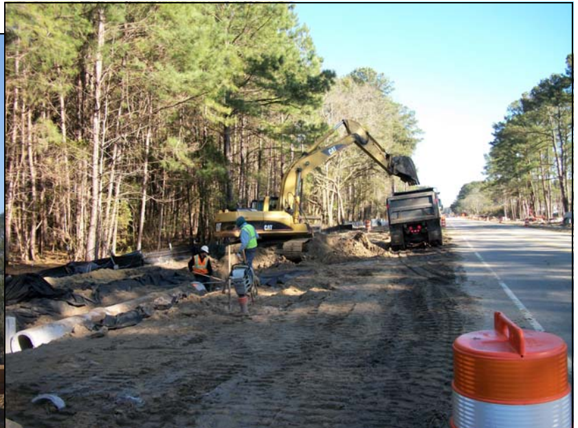
Pipe Crew Installing Storm Drain Lines Along Savannah Highway
