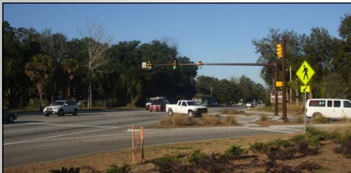
Realignment of the intersection of US 278 and Squire Pope Road with New Mast Arm Signals, which is Complete and Fully Operational
