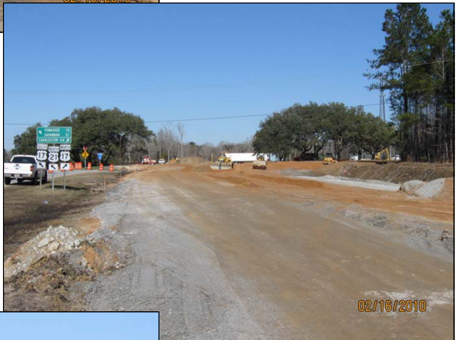
Building up the Embankment at Gardens Corner Intersection
