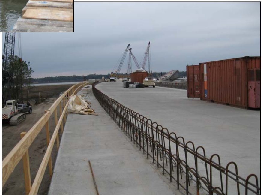
Pedestrian Walkway on the East End of the New SC 802 Bridge
