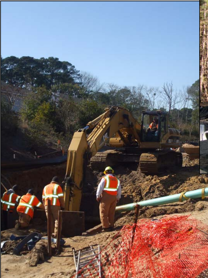
Utility Relocation Along Savannah Highway
