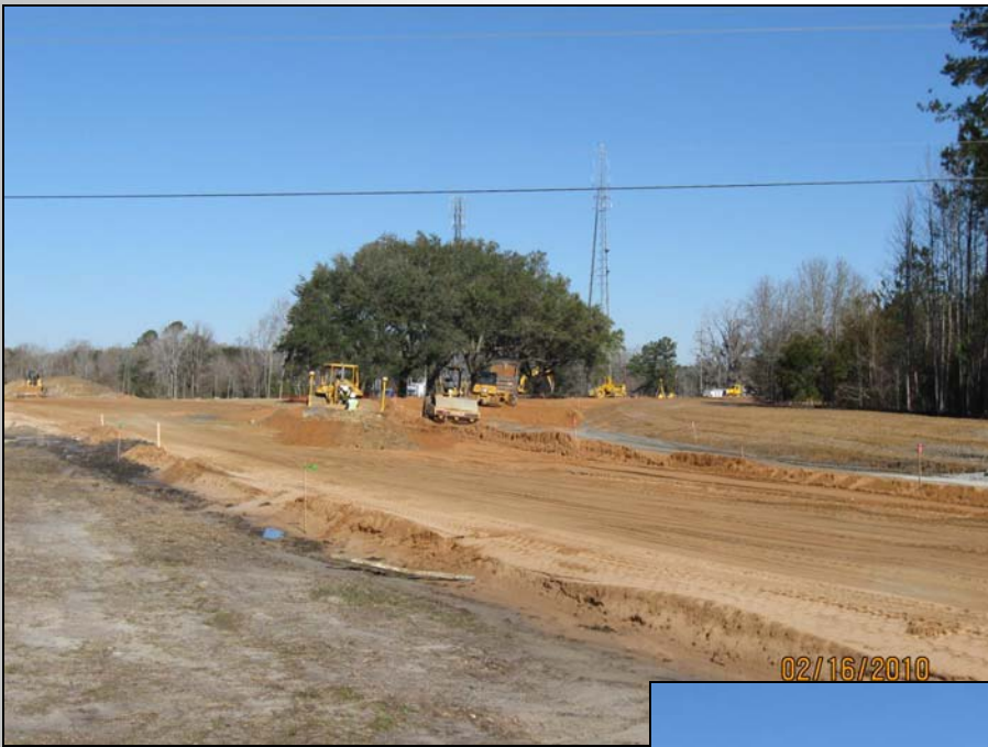
Building up Embankment for the US 21 / US 17 tie-in
