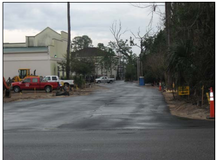
Completed Paving for New Frontage Road
