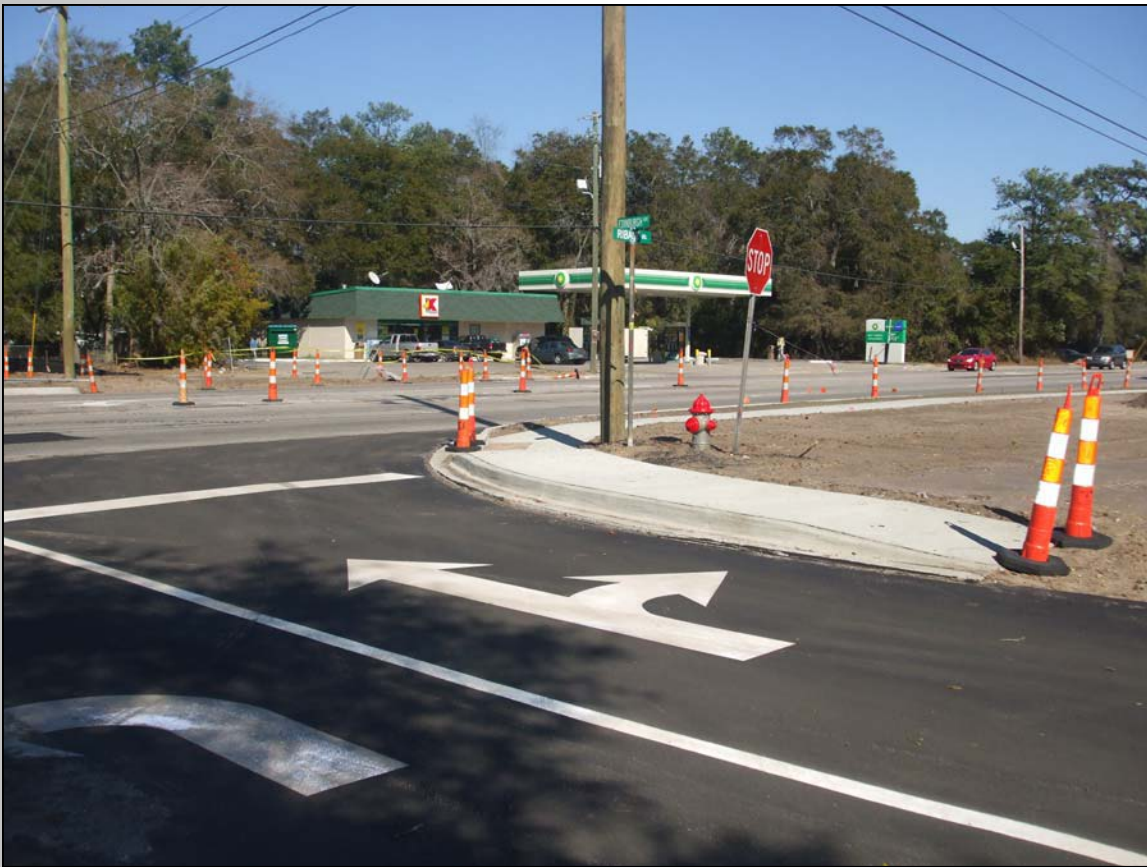
New Turn Lane and Sidewalk on Edinburgh Avenue
